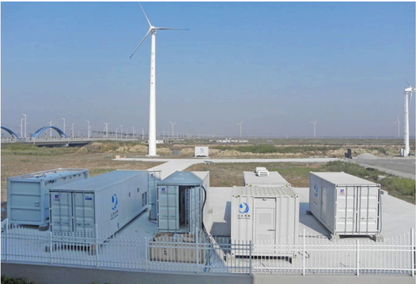
Seawater Desalination System
